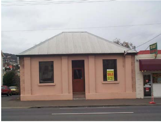
Figure 16 A Victorian Georgian former residence, 145 Davey Street. This structure is thought to date from the 1840s.
