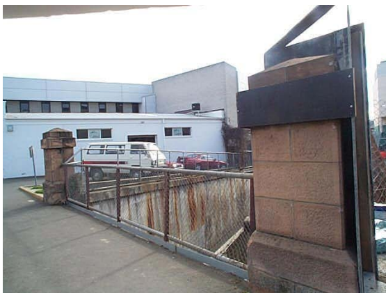
Figure 19 Sandstone pillars located on either side of Barrack Street, near the intersection with Collins Street. These are remnants of the Barrack Street Bridge that straddled the Hobart Rivulet from the early 1900s.
