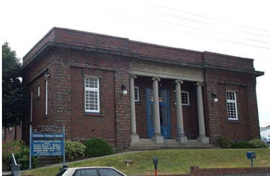
Figure 21 Christian Science Church at 69 Brisbane Street was designed by prominent local architect Bernard Walker, and constructed in c1929.
