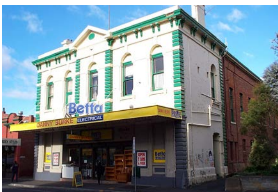
Figure 23 A shop at 52 Melville Street, which was constructed in 1890 as a Temperance Hall. It later became the Avalon Cinema, and functioned as such until 1976.
