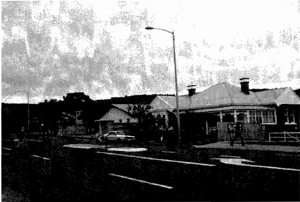
Issue ZB5 - 271-275 Sandy Bay Road beyond Chicken Feed store zoned Local Service under City of Hobart Planning Scheme 1982
