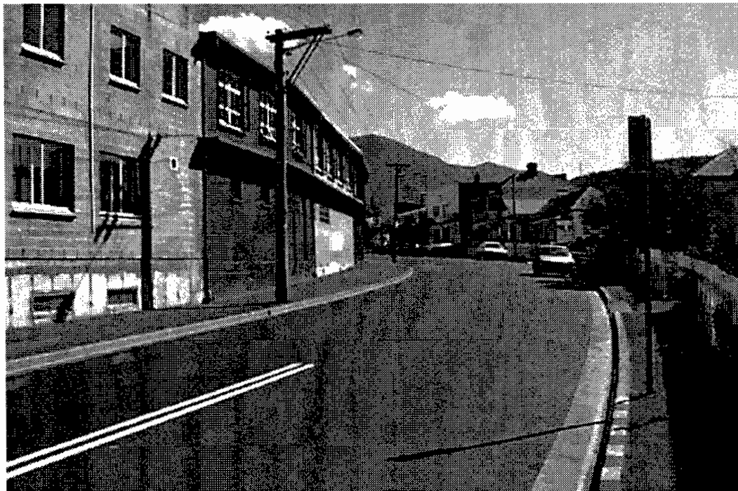
Issue ZB4 - Magnet Court one side of King Street; houses on the other provide the boundary of Zones 1 and 3 under the current Battery Point Planning Scheme 1979
