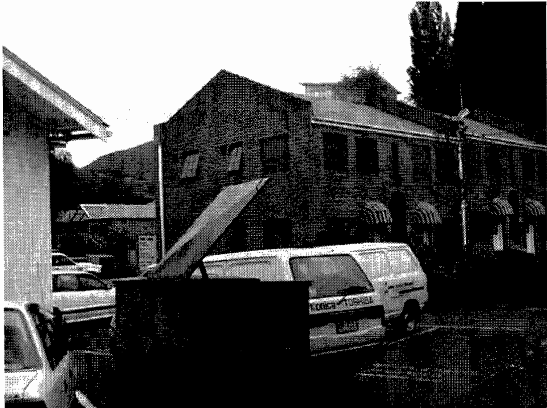
Issue ZB8 - Access to Bay Hire which along with visible part of Woolmer's Inn is within the residential Precinct 27, under the City of Hobart Planning Scheme 1982
