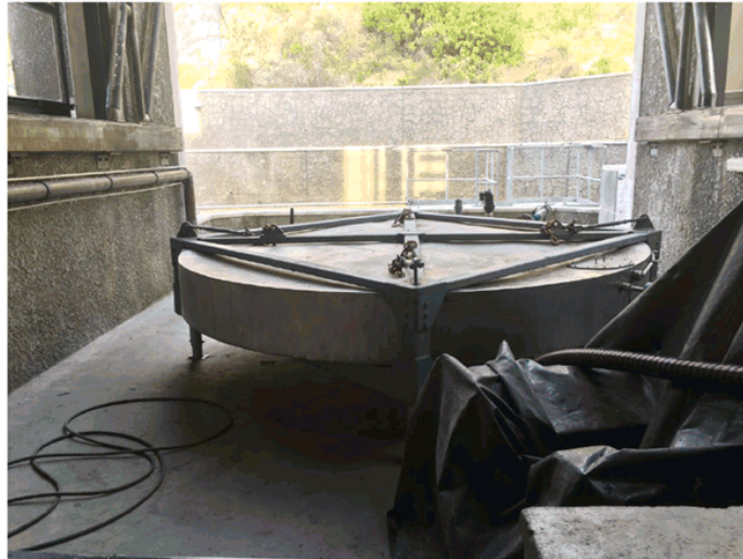
Figure 3: Wastewater Delivery Tank as used at Table Mountain Cable Car, Cape Town South Africa
