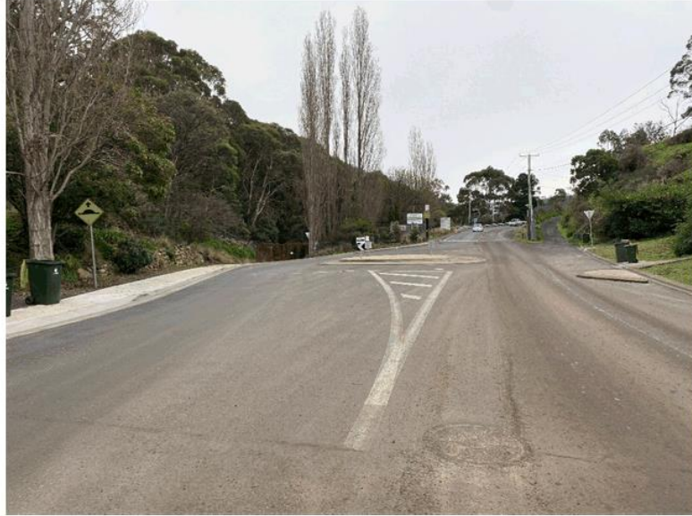
Photo 1: View towards McRobies Road roundabout and access road entrance.
