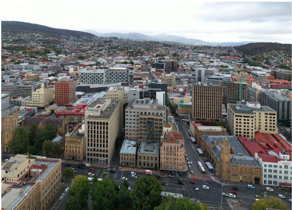
Aerial view of Macquarie and Elizabeth St and Central Precinct of Hobart. (Image source: Photographer Natasha Mulhall)
