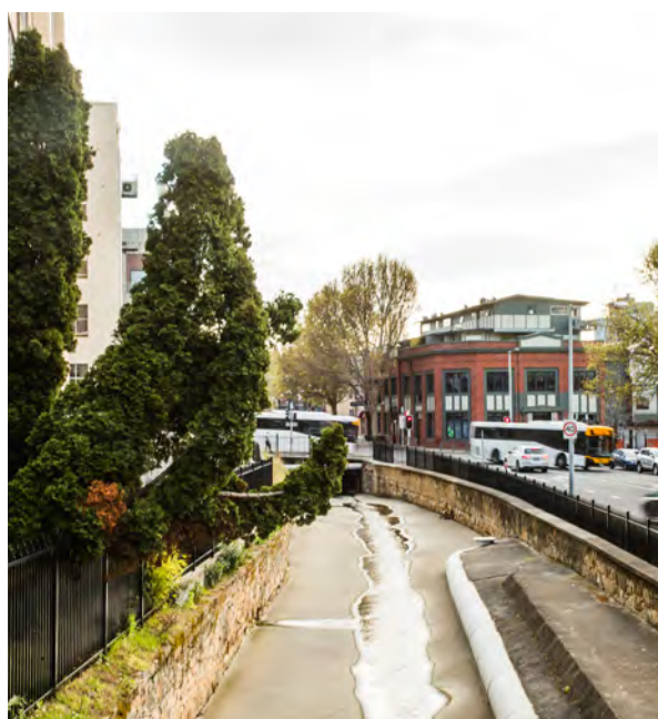
View of Hobart Rivulet along Collins Street (Image source: Photographer Natasha Mulhall)
