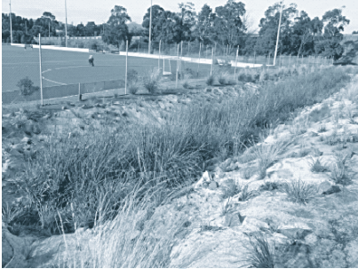
Bioretention swale [source: Melbourne Water]
