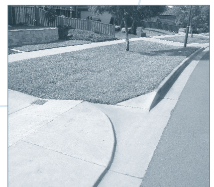
Grass swale in Lynbrook Estate, Melbourne. Curb 'funnels' direct road runoff into the swale system.
