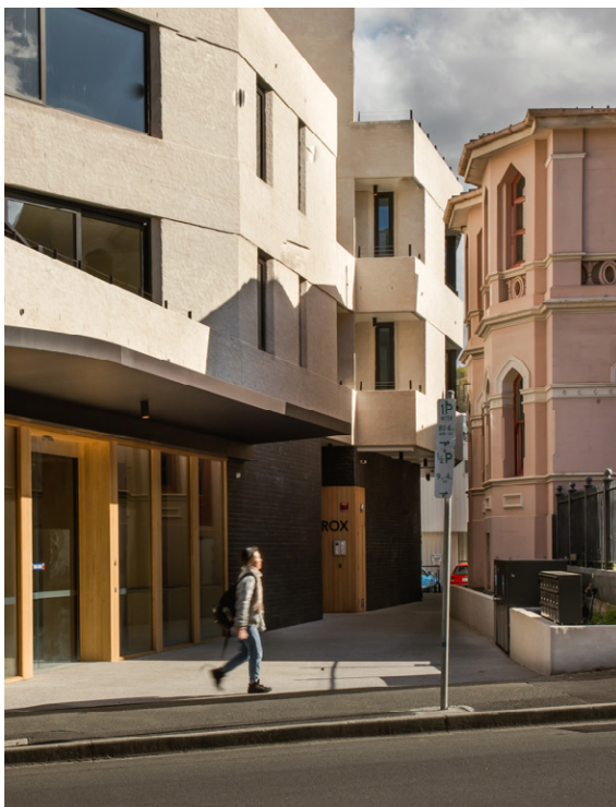
The Rox development on Elizabeth Street and its relationship to the existing on-site heritage building
