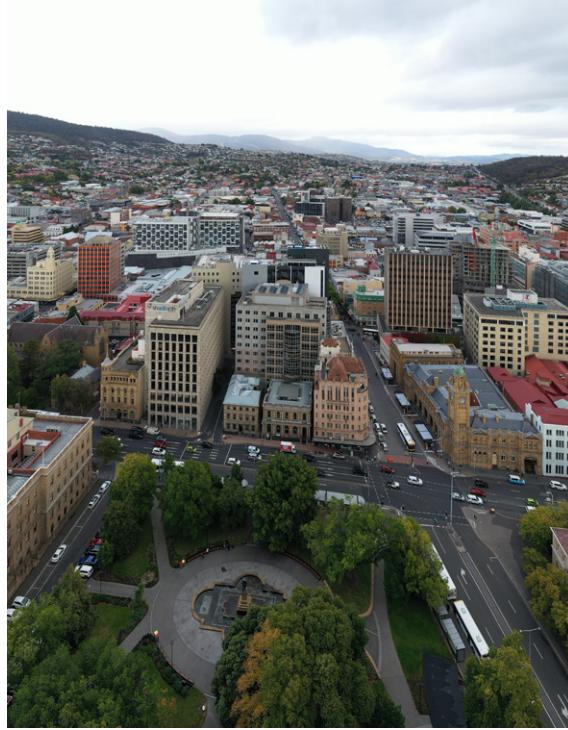
Aerial view of Franklin Square Photograph: Natasha Mulhall
