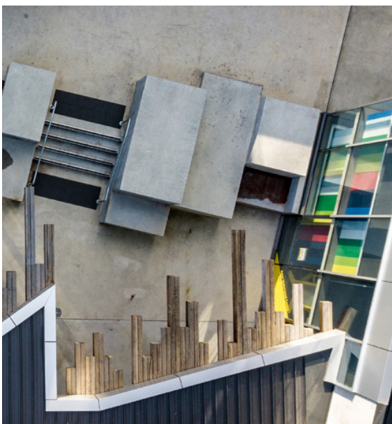
Aerial view of the internal courtyard of UTAS student accommodation Hobart Apartments
